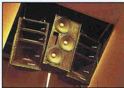
Two custom trapezoidal cabinets flank a custom bass cabinet in the main cluster.
