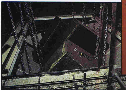
The main cluster is suspended through the ceiling in a cutout lined with Sonex, which keeps rear reflections to a minimum. Fiberglass batting was added to the rear of the loudspeaker cabinets. A grille covers the cluster and blends with the ceiling.
